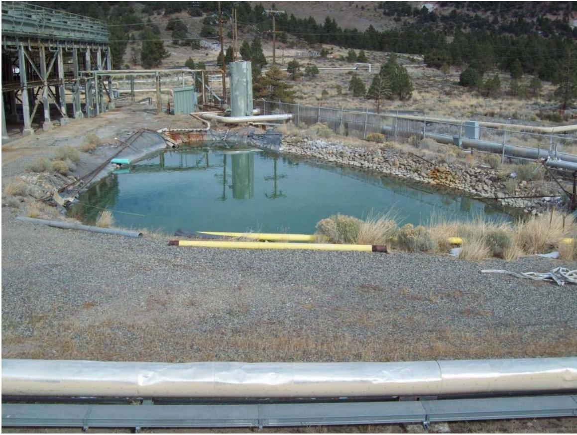
Figure 6. Fire safety pond (stored geothermal fluid, or “brine”) at MP-I power plant decommissioning area. Non-native grasses and rabbitbrush have colonized some of the disturbed habitat above the ordinary high water mark. The aquatic area does not support biological resources due to high salinity.
