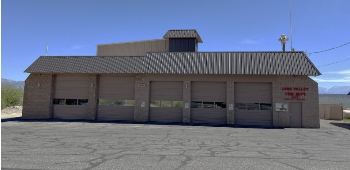
Figure 6: Existing LVFPD station in Crowley Lake
