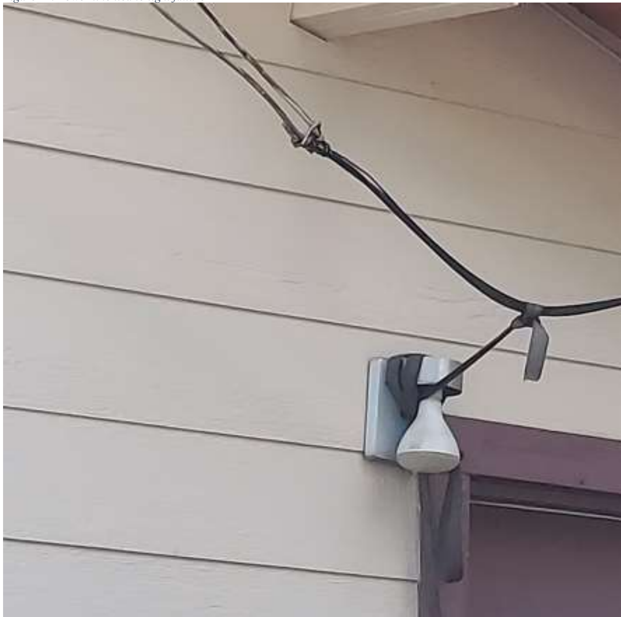
Figure 11. Power line tied to light fixture
