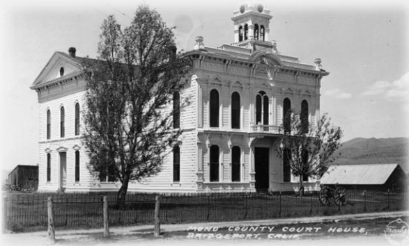
Mono County Courthouse 1920s
