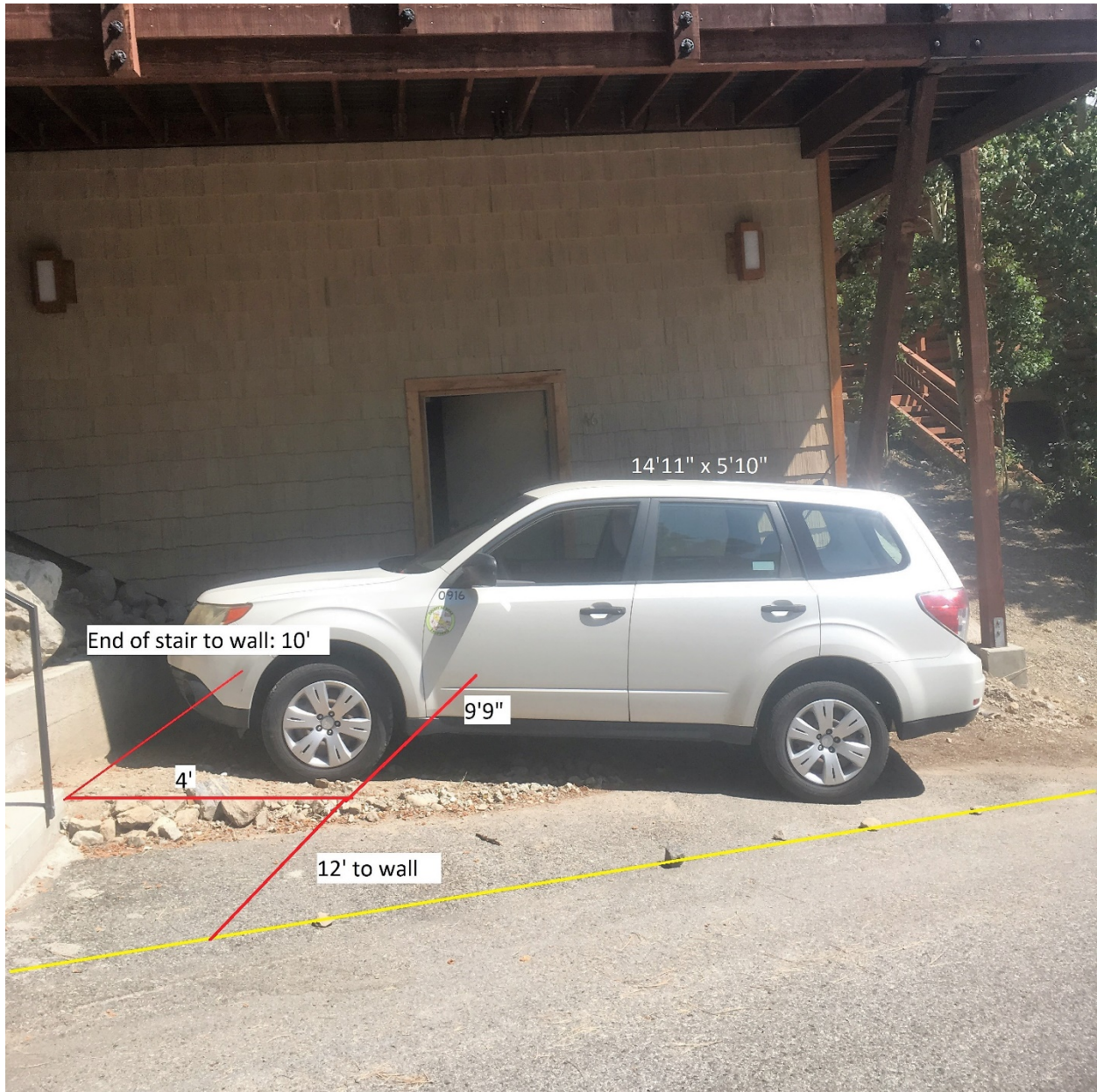
Figure 5: Additional measurements of parking area 1
