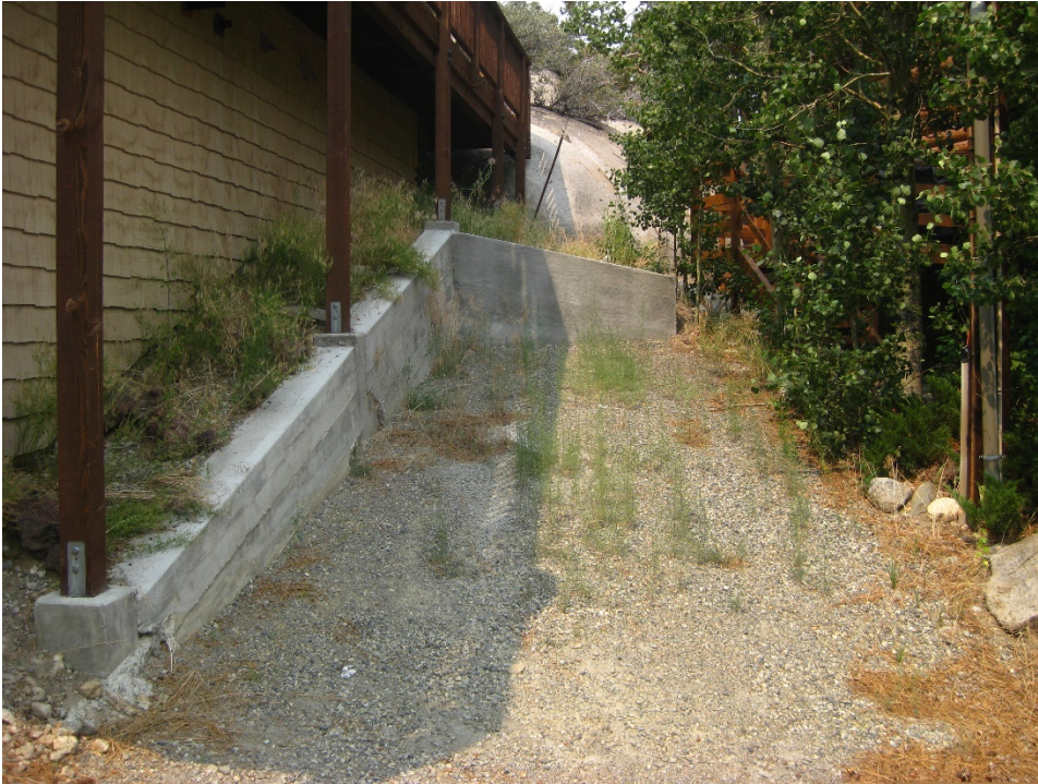
Figure 3: Side parking area 2
