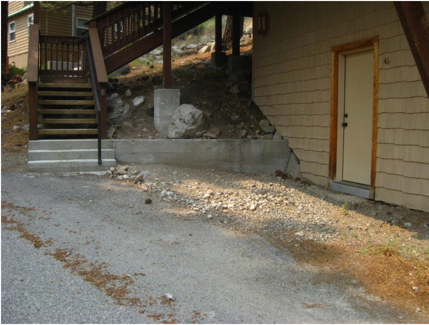
Figure 2: Front parking area 1.
