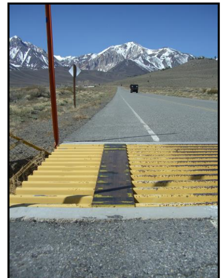
FIGURE 2. Example of Bicycle-friendly Cattle Guard on Benton Crossing Road.
