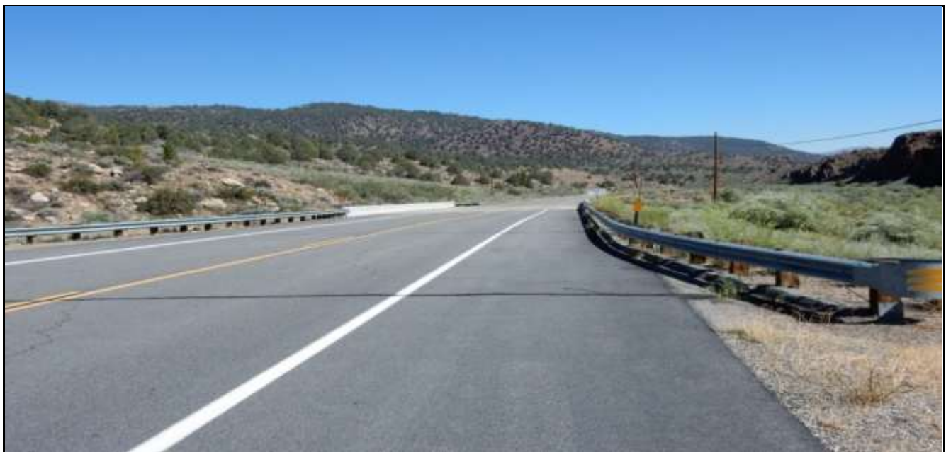
East Walker River Bridge at PM 6.20
