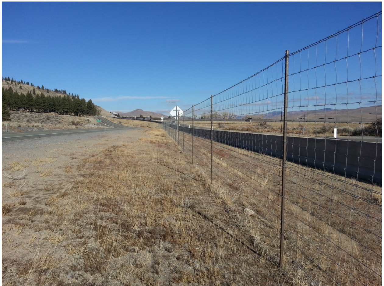
EXAMPLE DEER FENCE ALONG I-580 NEAR RENO – NOTE DARK COLORED FENCE POSTS
