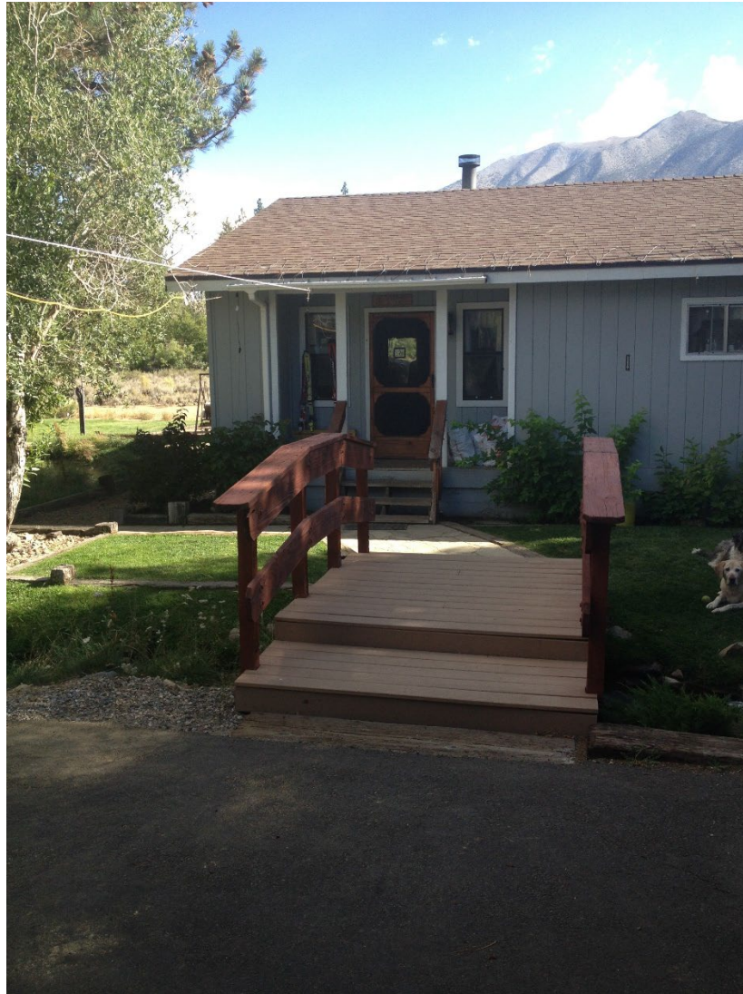
FIGURE 2: EXISTING FRONT ENTRYWAY
