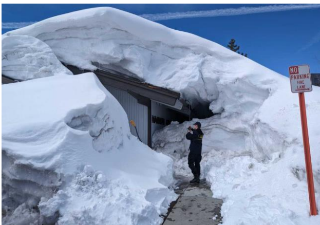
Figure 6: Responder conducting a building and structural inspection.
