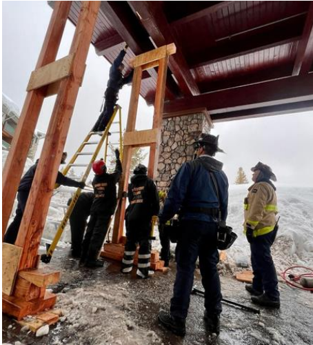
Figure 1: Urban Search and Rescue (USAR) team adding structural support to a building.
