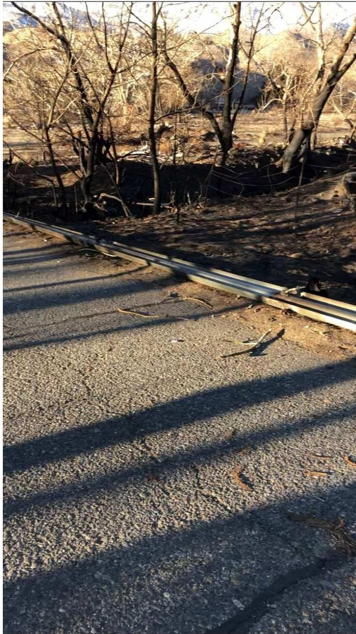
Photo 4 – North River Lane Guardrail. Westbound lane protecting from irrigation canal that crosses under road.
