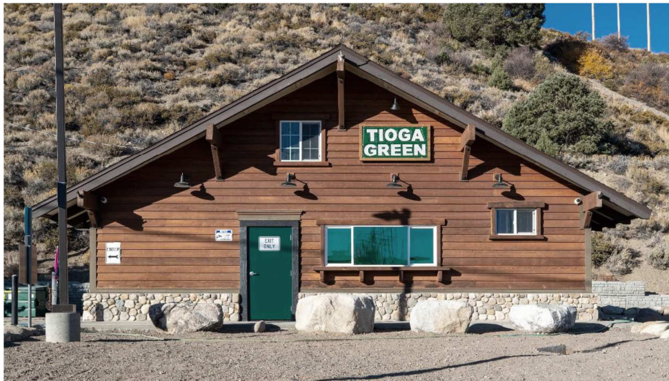
Figure 2: Existing sign (12-square feet).
