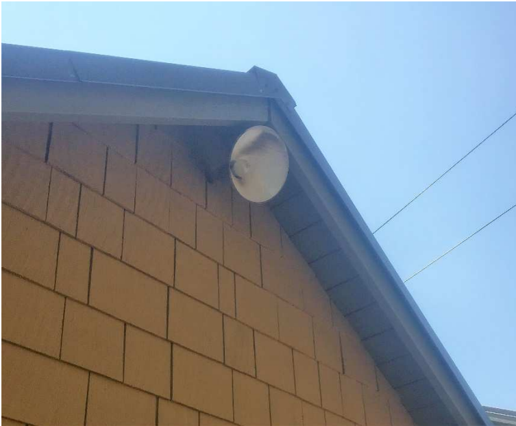
Figure 5 Rear lighting; light shield does not adequately prevent light trespassing
