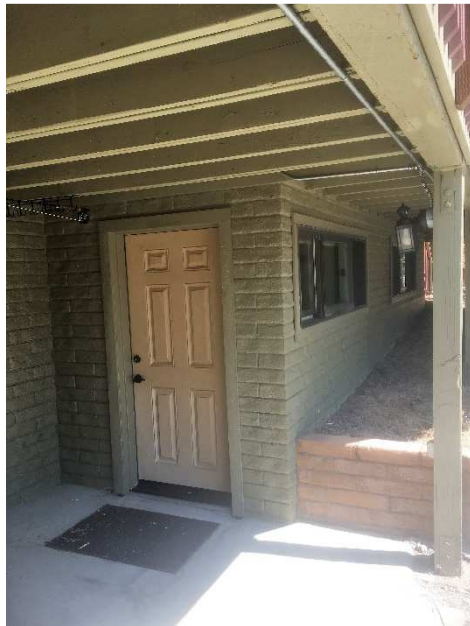
Figure 4: Secondary entrance lighting
