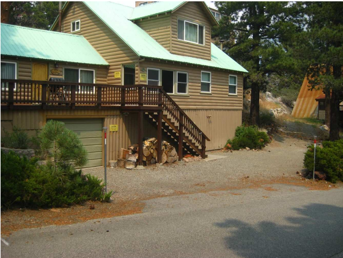
Figure 2: Addressing and parking need to be improved to meet General Plan and MCC standards. The structure also lacks snow guards above the main entrance and staircase.
