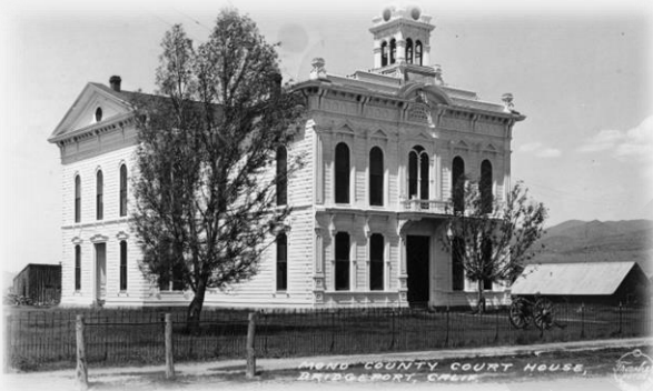
Mono County Courthouse 1920s
