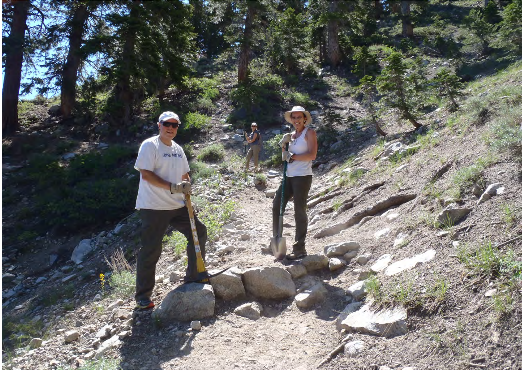
Figure 7. Volunteers Roland and Marni Wieshofer repairing a waterbar on the Fern Lake Trail (photo by Julia Runcie).
