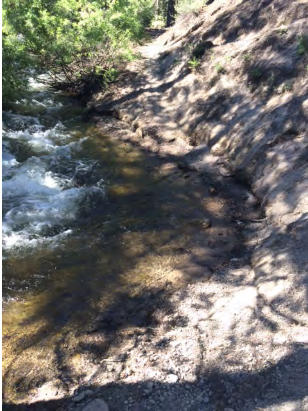
Figure 10. Washed-out section of the Glass Creek Meadow Trail (photo by Astra Lincoln).
