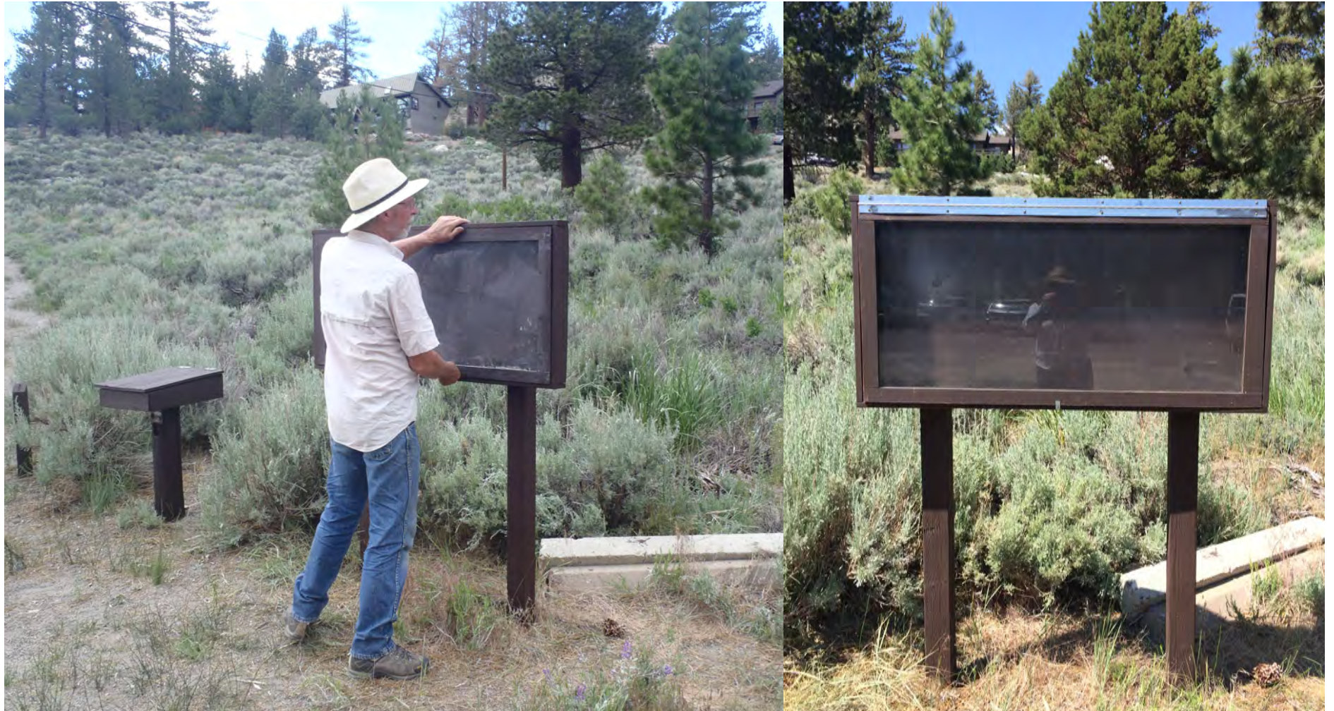
Figure 5. Volunteer Jim Wells of Snowflake, AZ and June Lake repairs the Gull Lake trailhead kiosk (photo by Julia Runcie; the finished product (photo by Jora Fogg)).
