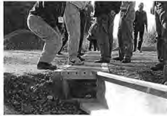
Fig. 1. Amphibian tunnel for mitigating road mortality (Federal Highway Administration, 2002).
